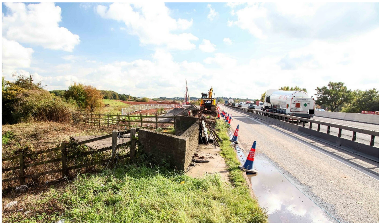
Figure 5-4 Derwent Valley Aqueduct (Warren Farm Culvert) SB with earthworks widening under construction
