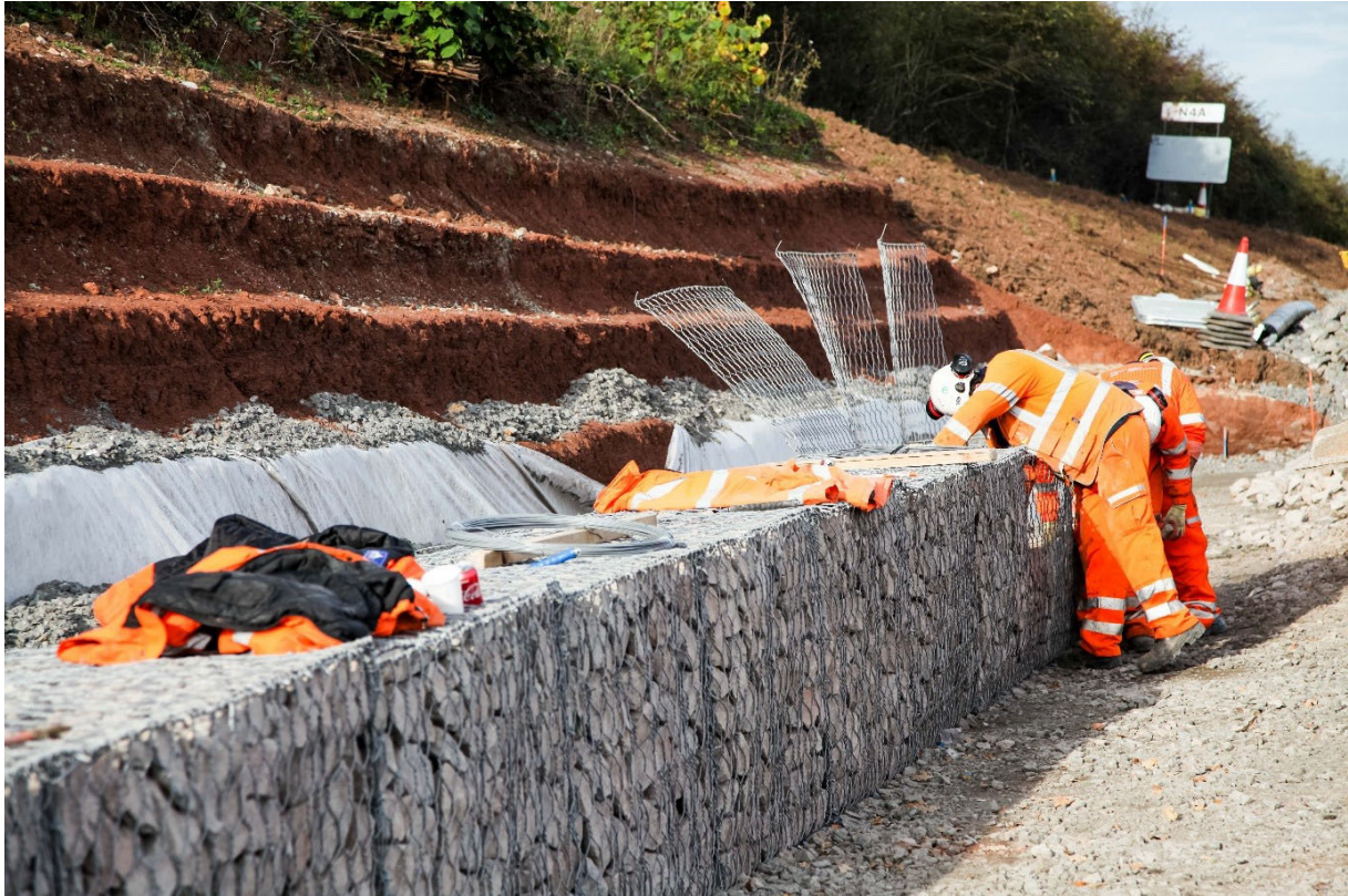
Figure 5-6 Gabion wall construction CH 182800 - detail
