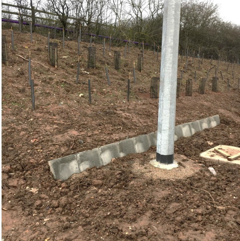
Figure 5-8 Typical slab-on-edge wall at minor structure location
