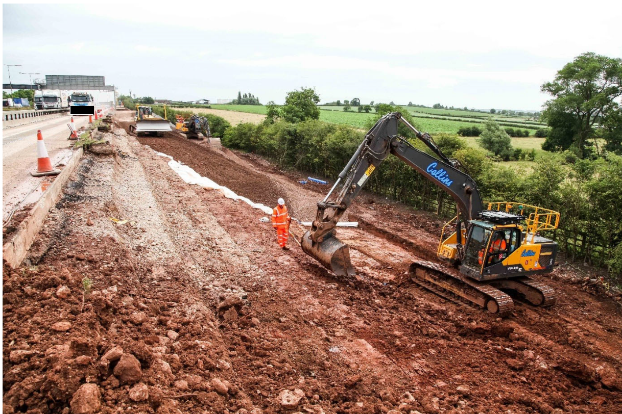
Figure 4-1 Typical embankment widening construction at CH 183100 SB
