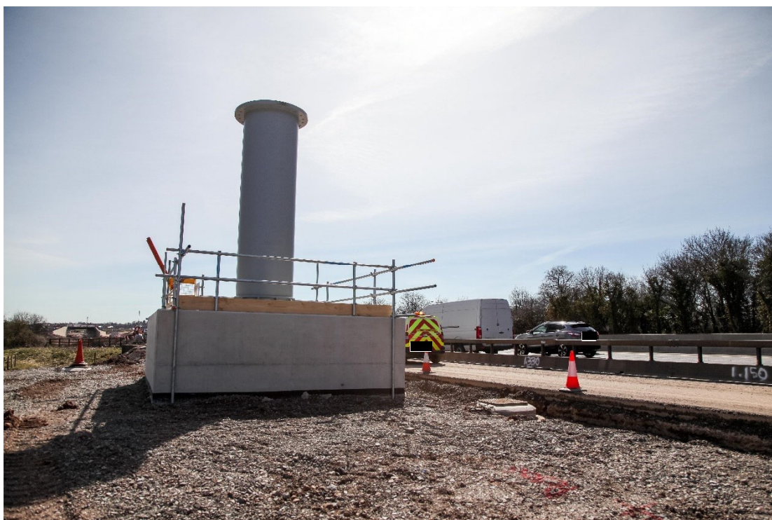
Figure 10-3 Completed 2x2 pile cap Gantry G203
