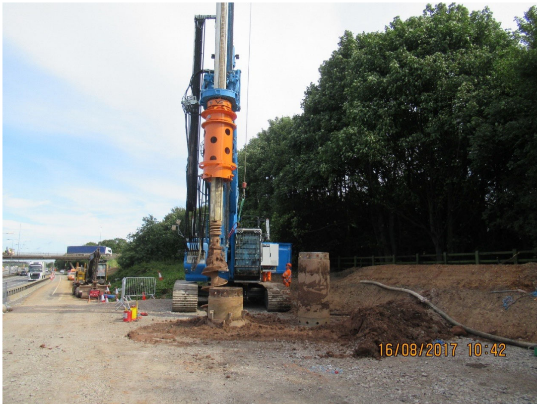
Figure 10-2 900mm diameter pile installation using Soilmec SR-75 rig
