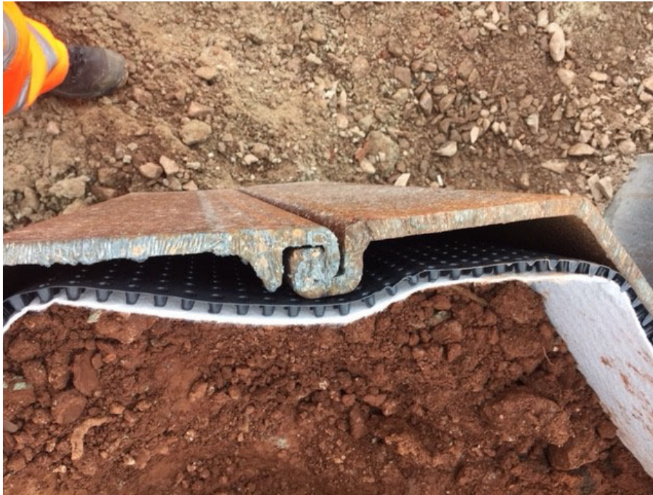
Figure 5-2 Deckdrain layer behind backfilled sheet piles in cuttings
