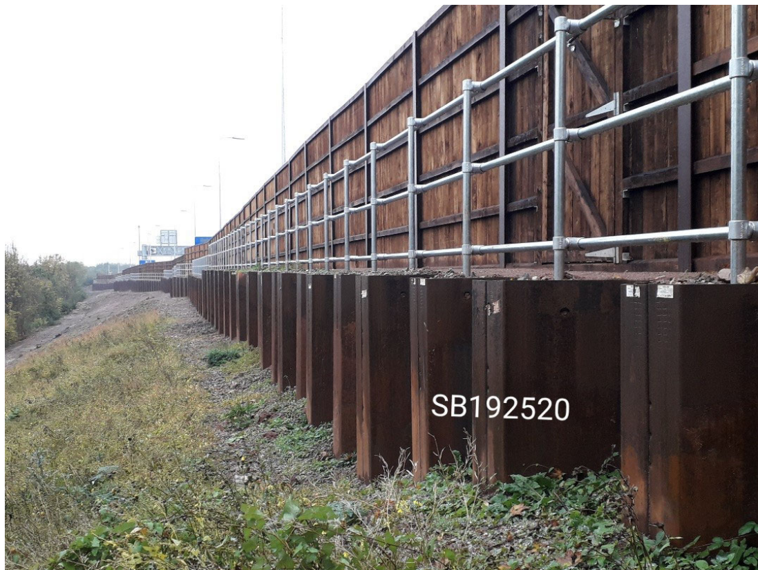
Sheet Pile Wall at SB192520
