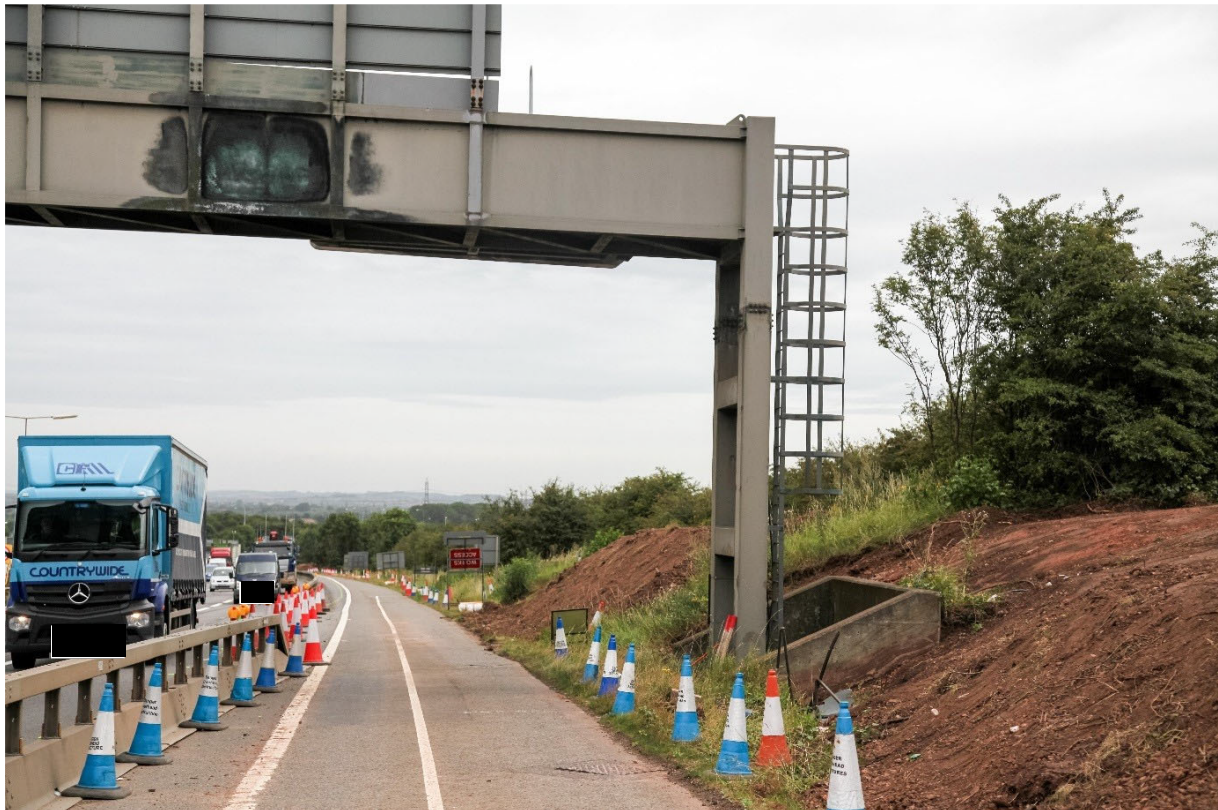
Figure 3-1 Typical minor regrade to cutting slope around existing gantry G111 SB
