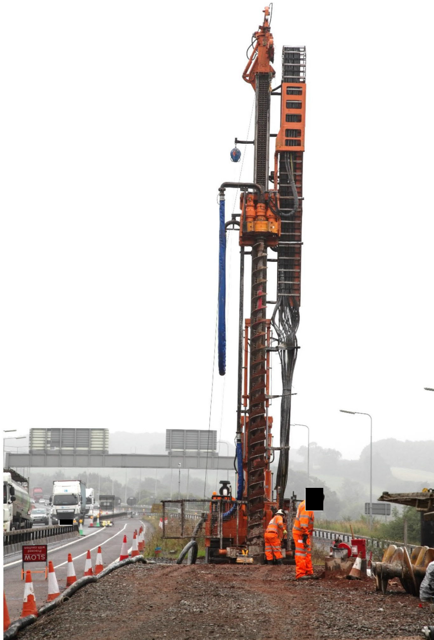
Figure 10-4 750mm pile installation with Hutte rig (Gantry 318)
