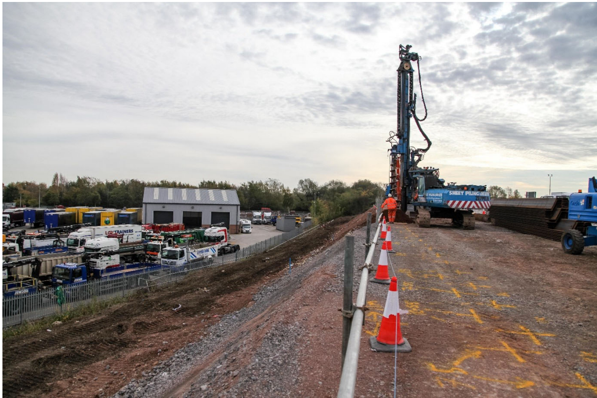
Figure 5-3 Sheet piling on embankment at ERA E3-B1
