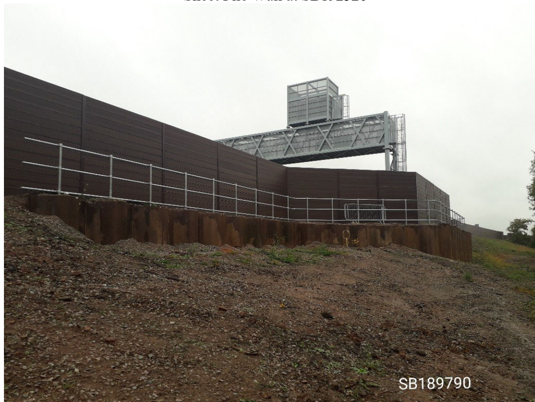
Sheet Pile Wall at SB192520
