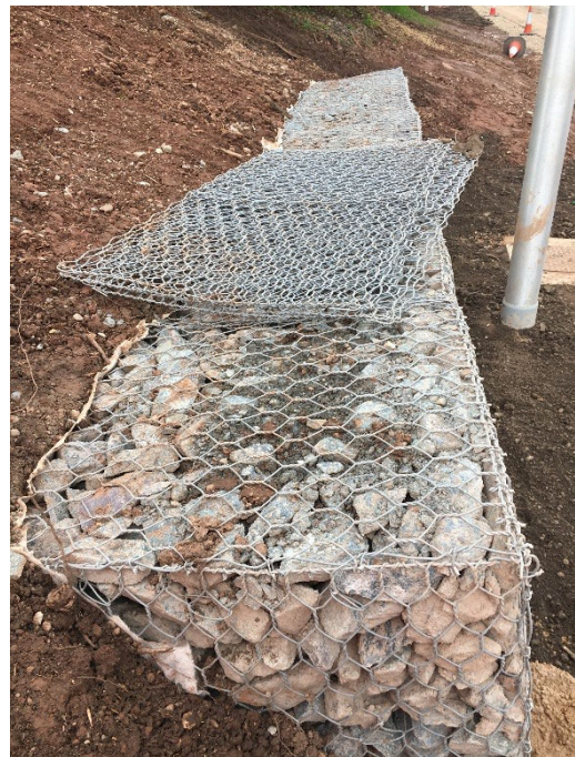
Figure 5-7 Small gabion wall behind lighting column
